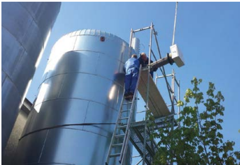
Figure 11: Delivery of thermal energy storage and assembly of heat elements [Rothmoser]
