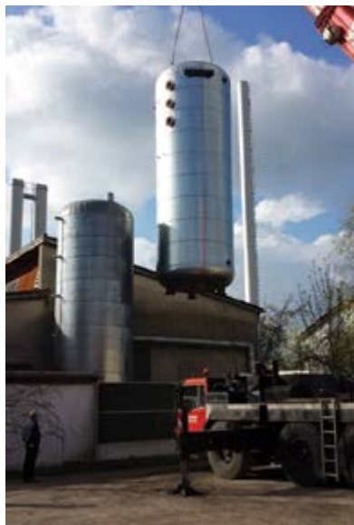
Figure 11: Delivery of thermal energy storage and assembly of heat elements [Rothmoser]
