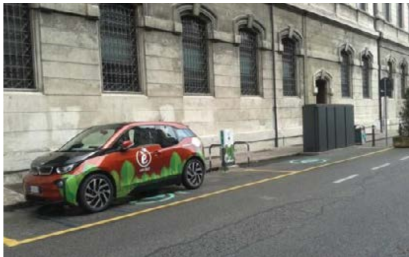
Figure 5 - The AlpStore Mantua Pilot: car, charging station and the technical cabinet with switchboard, plc, power meters, modem router, UPS and battery
