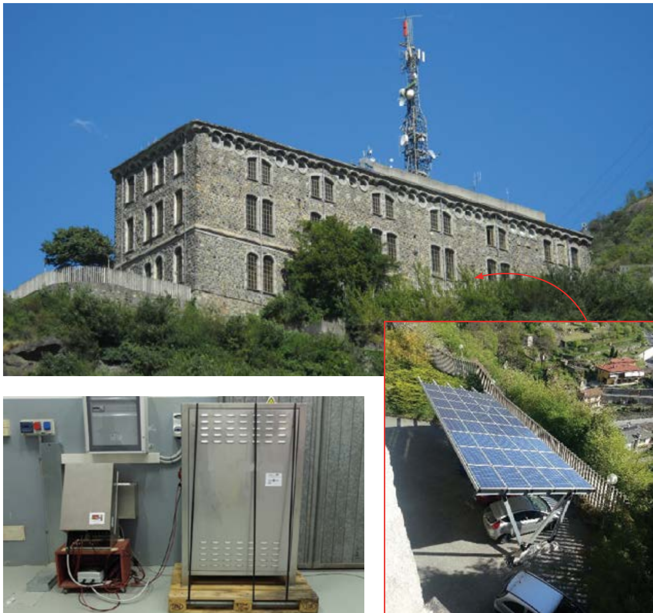
Figure 1 –The Smart Node Pilot Project Building (above) the power converter and the storage (bottom left) and the PV system (bottom right)
