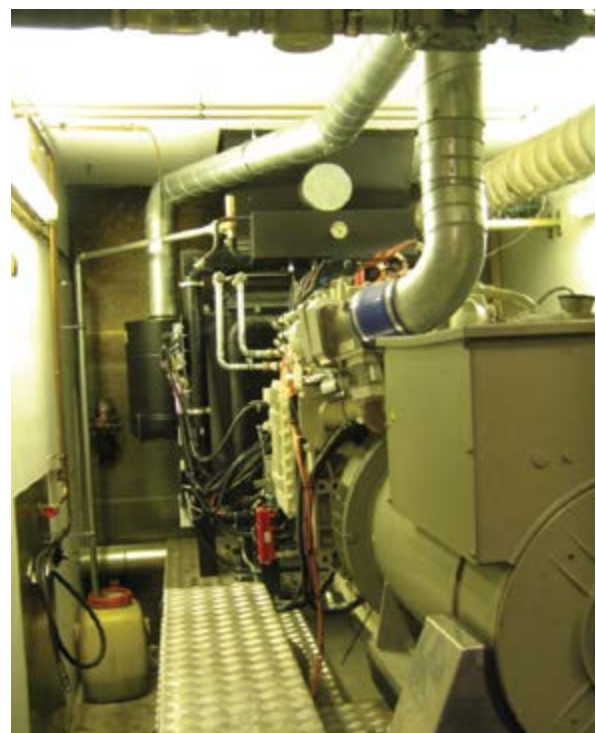
Figure 9: Existing thermal energy storage system in Grafig (left side) and CHP unit (right side) [FfE]
