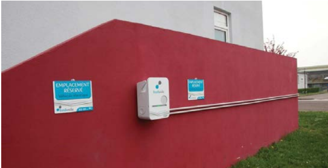
Picture of the first site in Entzheim, with a 22-kW charging station and two dedicated parking spots
